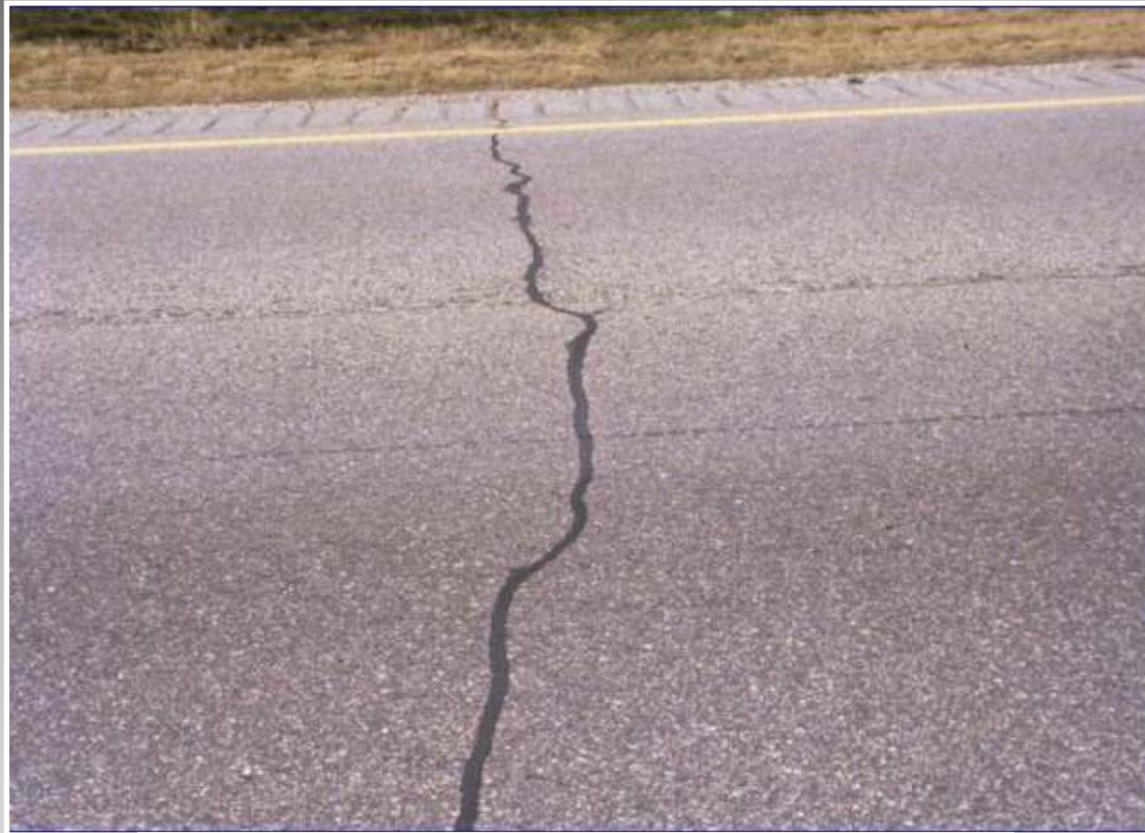
Sealed Transverse Crack
